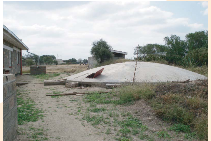
3. An underground tank for rainwater off Kajiado's rooftops.
