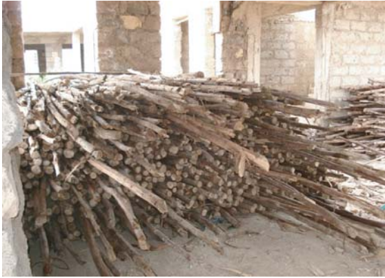
1. Wooden scaffolding poles.
