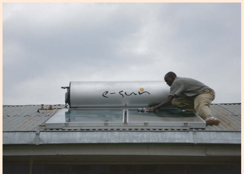
4. fixing a passive solar water heater to a roof in Kajiado
